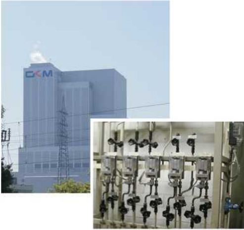
Lower picture shows 5x precision pressure switch MANOCOMB® model IP65 version 2KA/VAMG used in power plant "Grosskraftwerk Mannheim (upper picture).
